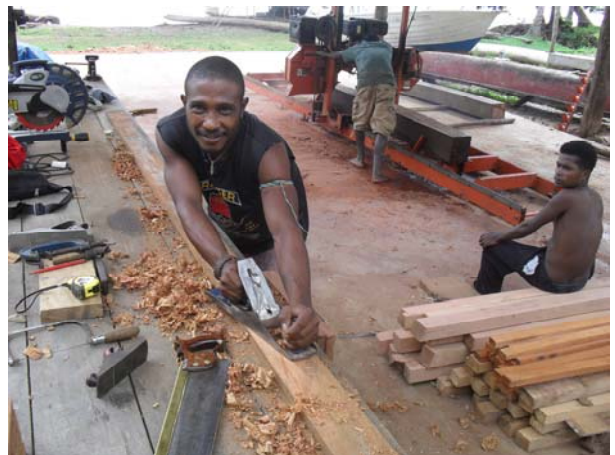
Abi constructing student benches with tools donated to us by Tools for Self Reliance
